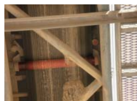
Conveyor belt idler
